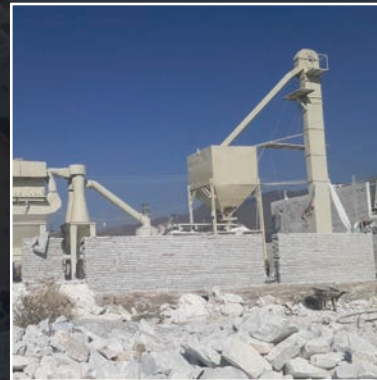
Limestone Grinding Plant
